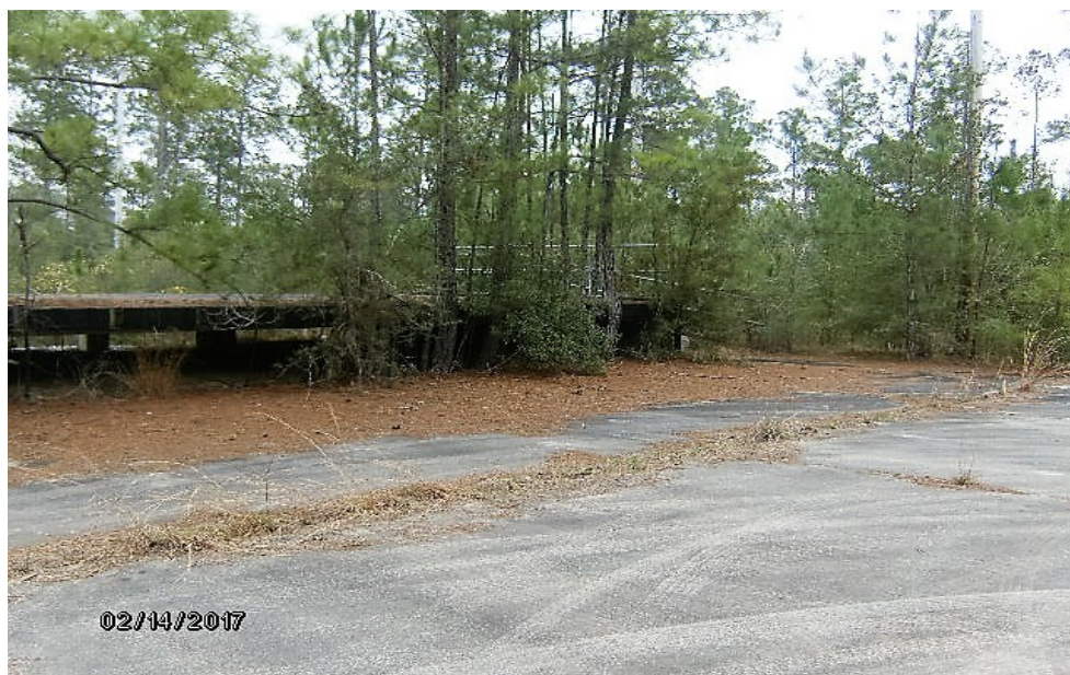
Figure B-4. The former Suspect Car Control Loading Area used during MSAAP operations located within Area A.
