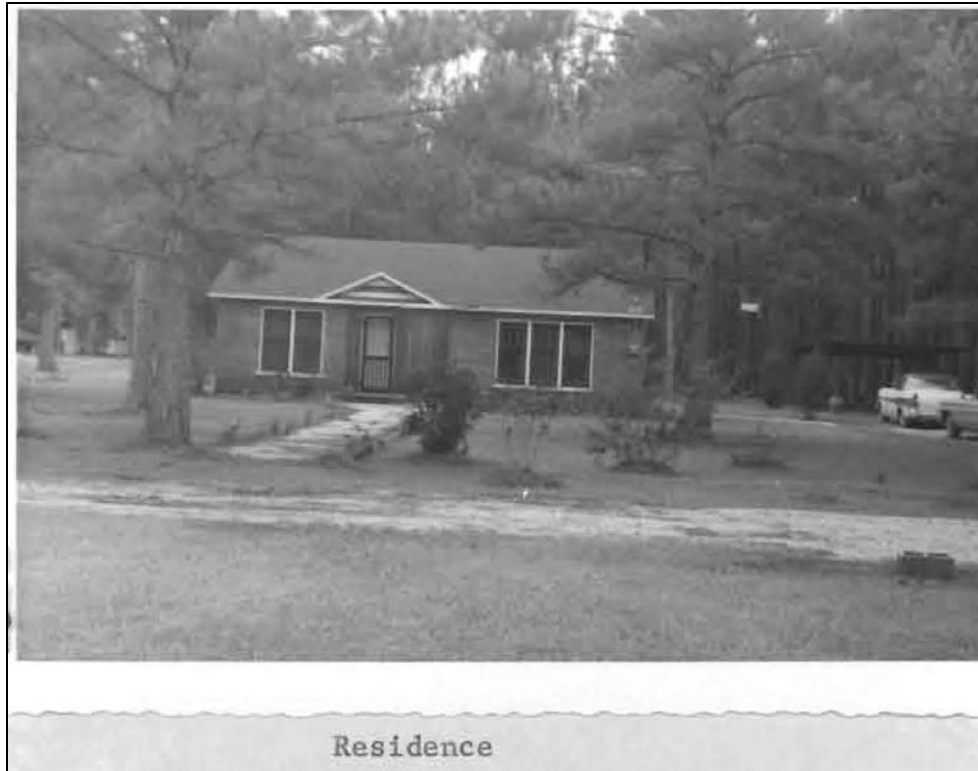
Figure 18. Structure in Tract 238, possible correlate to 1957 topographic structure.
