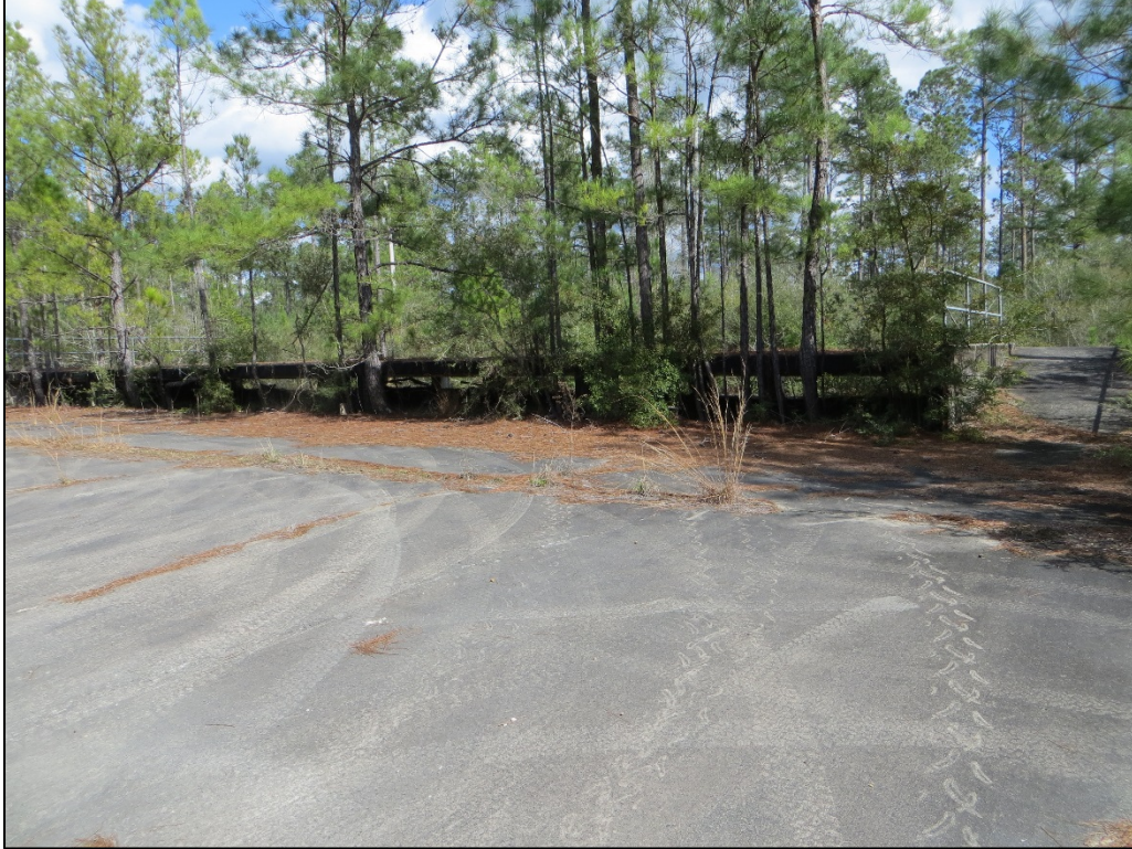
Figure 23. Looking east at the concrete pad and loading station.
