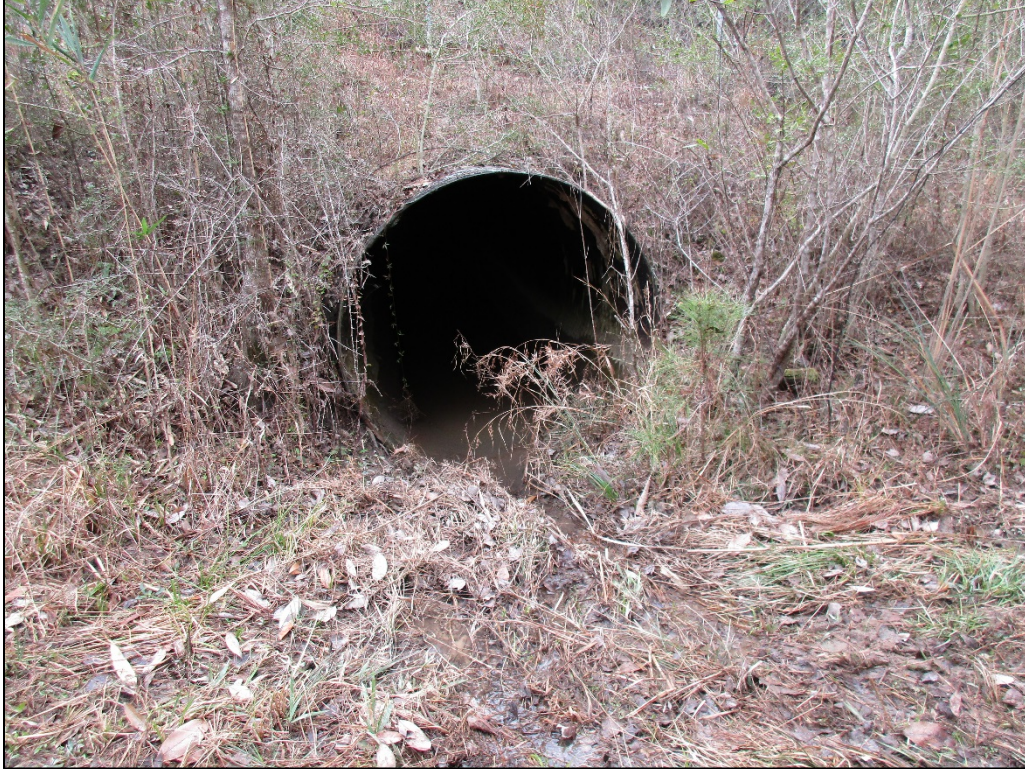
Figure 26. Example of culvert in Parcel A.
