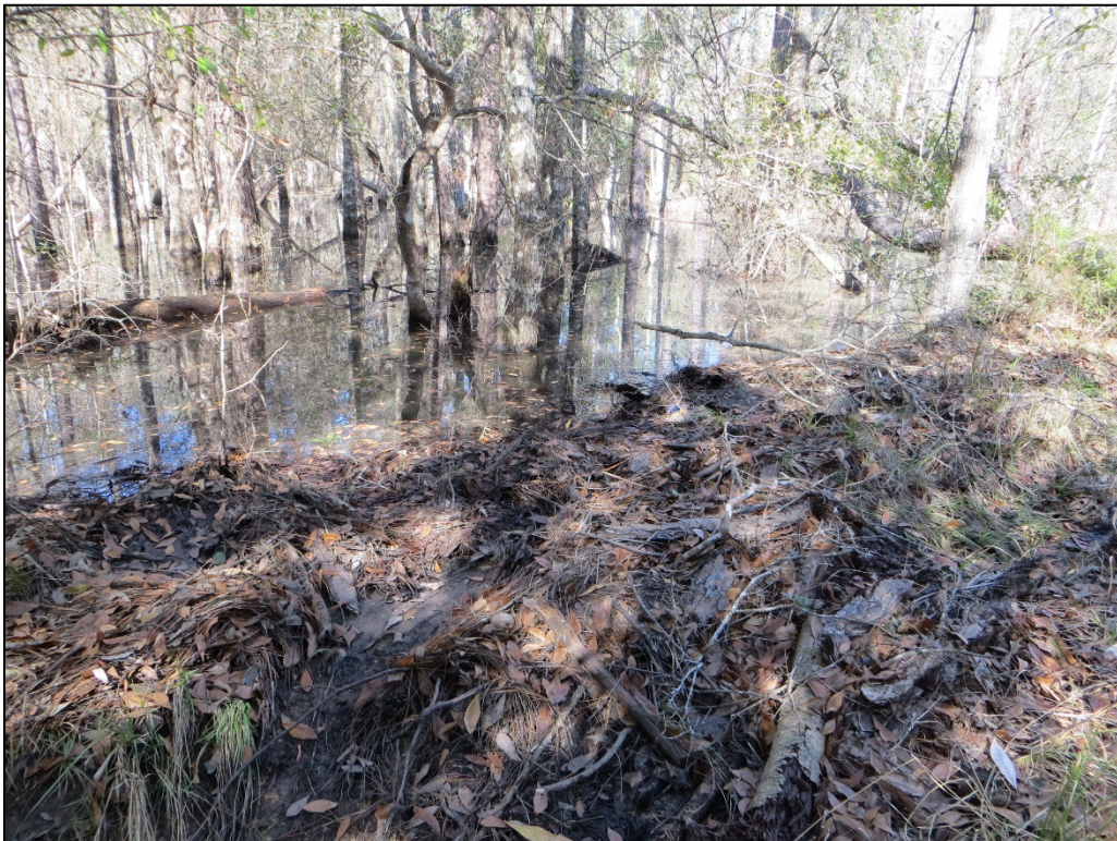
Figure 8. Edge of floodplain in southeast portion of Parcel B, earthen embankment and drainage pipe present.
